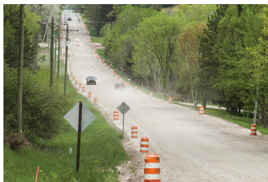
Construction in progress on Marion Center Road. Photo by Karen Walker.
